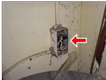
7.3 Picture 6 Storage room
