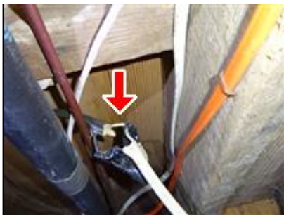
7.3 Picture 5 Storage room
