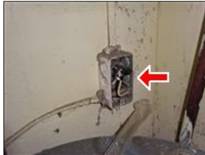
7.3 Picture 6 Storage room
