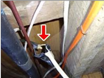
7.3 Picture 5 Storage room
